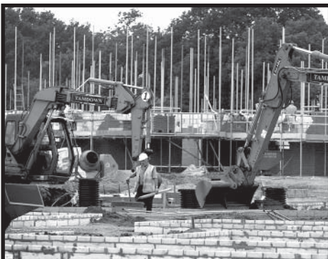
Development at Colchester Garrison
