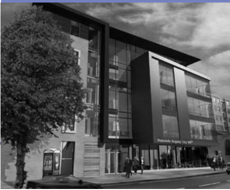
Westminister Kingsway College's £53.5 million redevelopment
