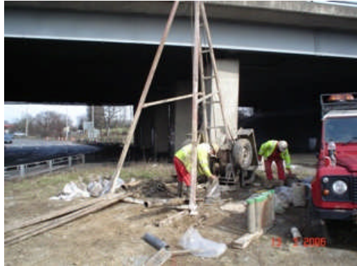
NVQ Land Drilling qualified drillers at work
